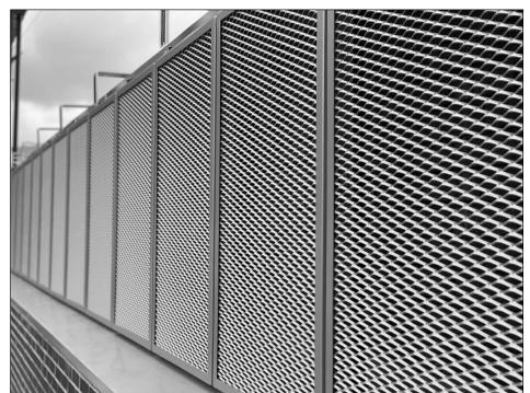
Lighting from vehicular headlights to be deflected down by the Mesh Cladding minimising Light Spill from Proposed Top Floor.
