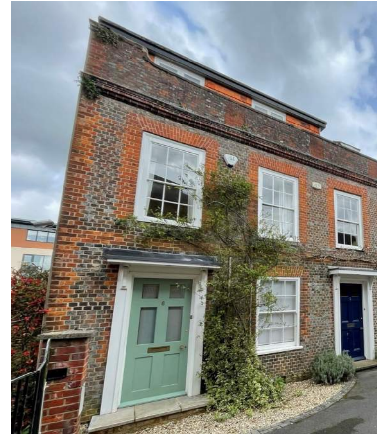
Figure 3.35: Listed Building with the benefit of a roof conversion and terrace.
