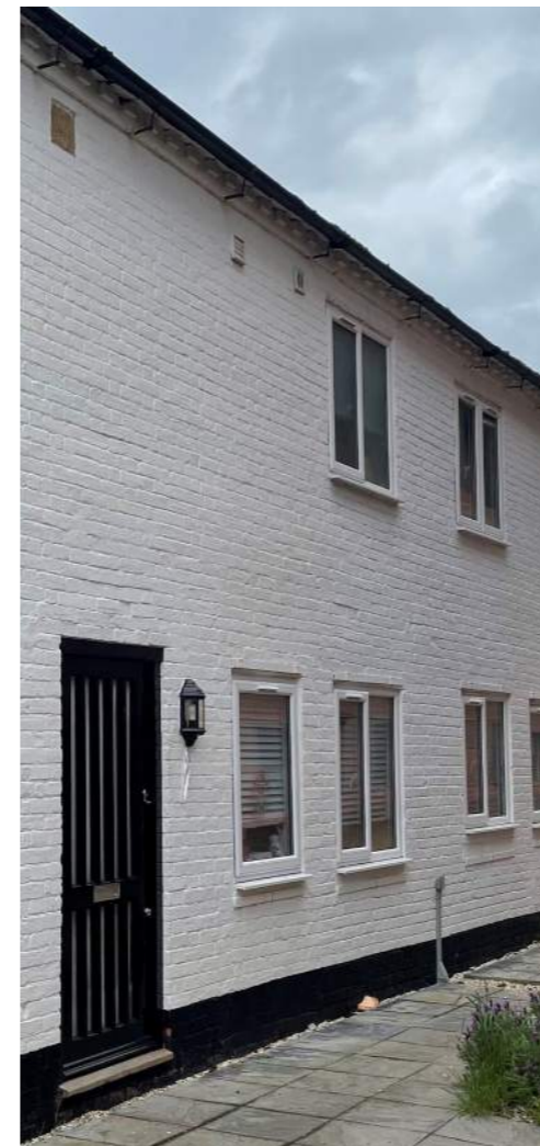
Figure 4.29: R/O Northcroft Street.
