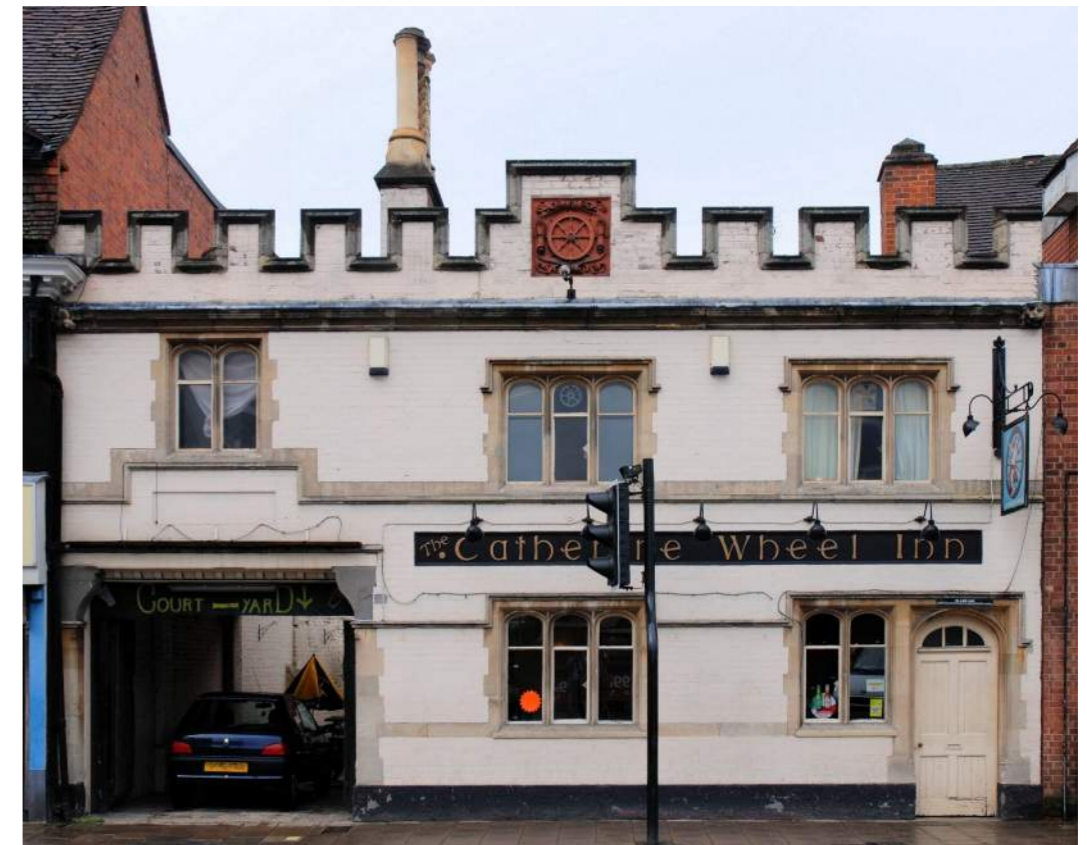
Figure 2.11: The Catherine Wheel Inn. (Source: Historic England).
