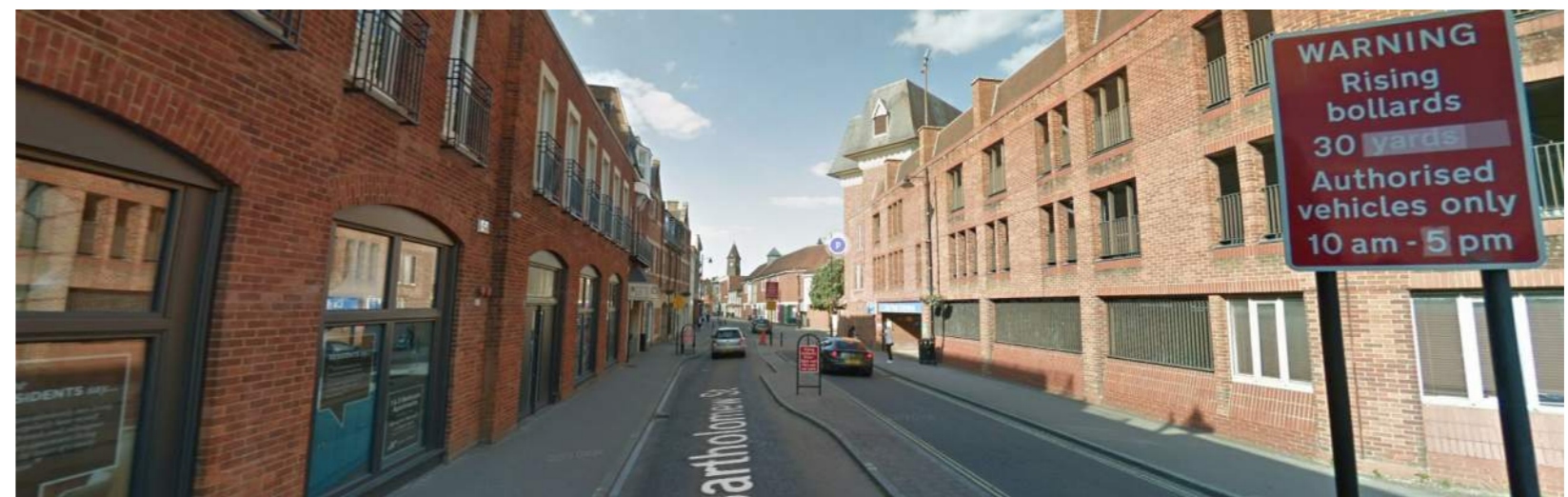
Figure 2.46: Bartholomew Street (South) has narrow pavements, some traffic restrictions and access to the Car Park which creates a different character and environment form the Northern extent of Bartholomew Street.
