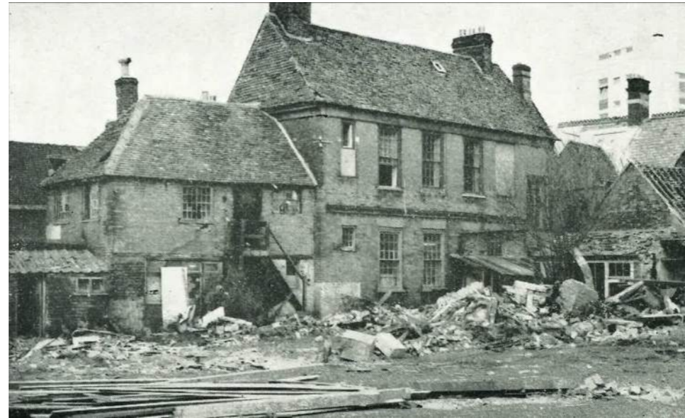
Figure 3.11: Accommodation Wing behind No. 25 Cheap Street, just before demolition.
