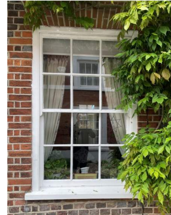
Figure 2.33: The use of semi-reflective glass is noticeable, which assists with privacy given the close proximity of threshold curtilage.
