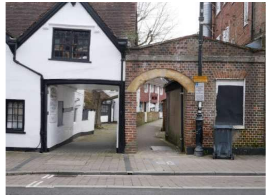
Figure 3.49: Eight Bells Carriage Arch and the adjacent Passageway Arch.
