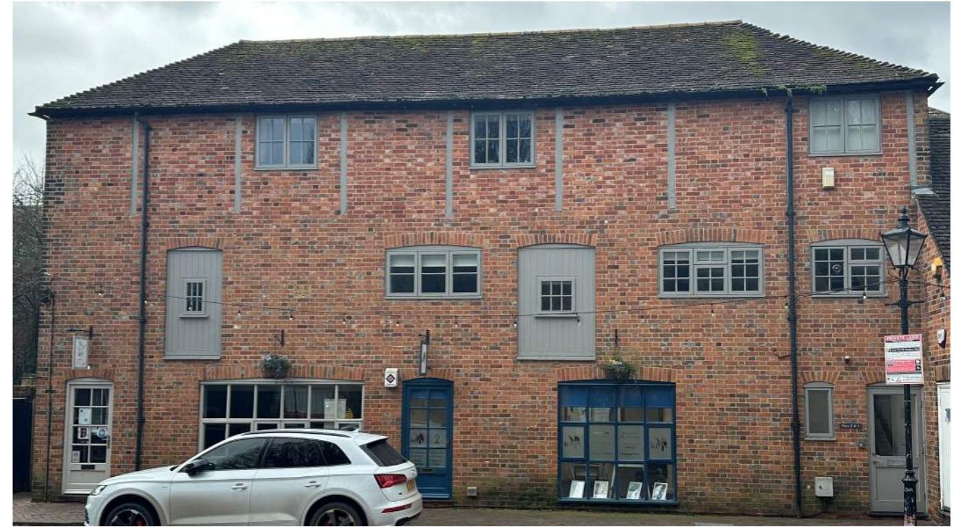
Figure 4.24: Inch's Yard, Market Street.
