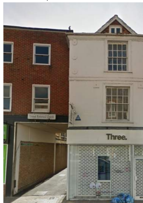
Figure 2.32: 80 Northbrook Street with passageway entrance to the left.
