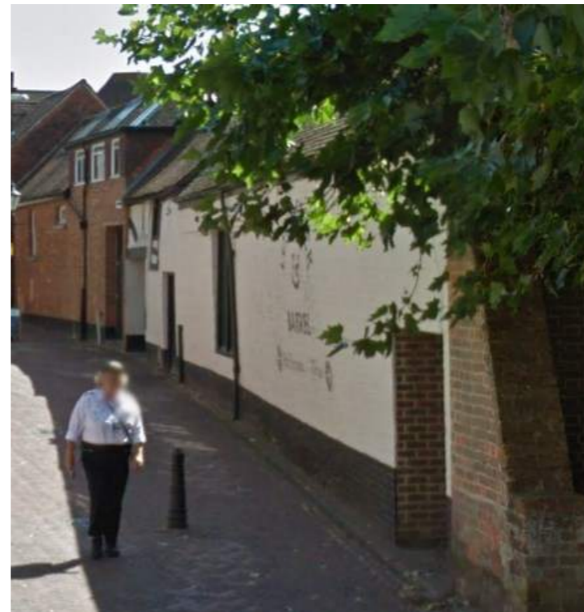
Figure 3.39: The r/o 103 Northbrook Street, the former stables, illustrates a traditional collection of materials and a interesting roofscape of diffing storeys, pitches and treatments.
