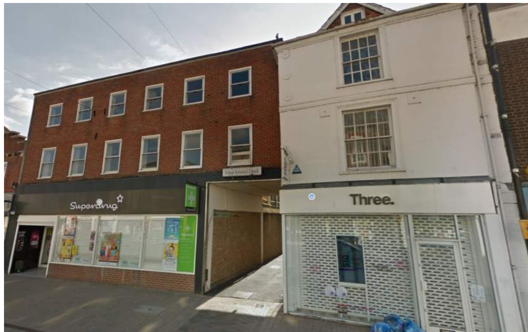
Figure 3.32: No. 81 Northbrook Street and the Passageway to Cromwell Place. No. 80 (Three) is Listed.
