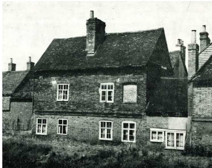
Figure 3.10: Vine Cottages, Bartholomew Street (demolished).
