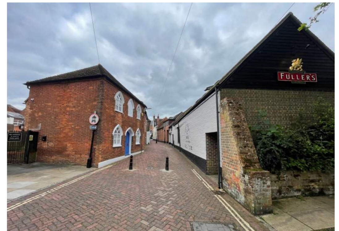
Figure 3.41: View from the West with the Almshouse to the left and the former stables to the right. A notable feature here is the gothic fenestration on the former and the buttress to the latter.
