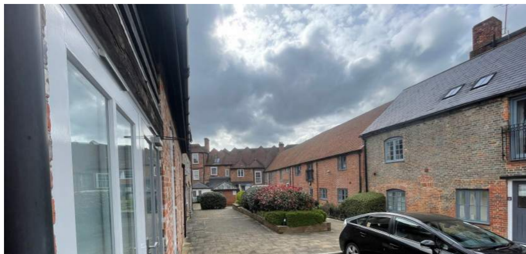
Figure 2.38: Outbuildings to the r/o 24 The Broadway (former Adnams Brewery) are on the left hand side with the outbuildings to the r/o 4 Oxford Street on the right frame the linear courtyard space.
