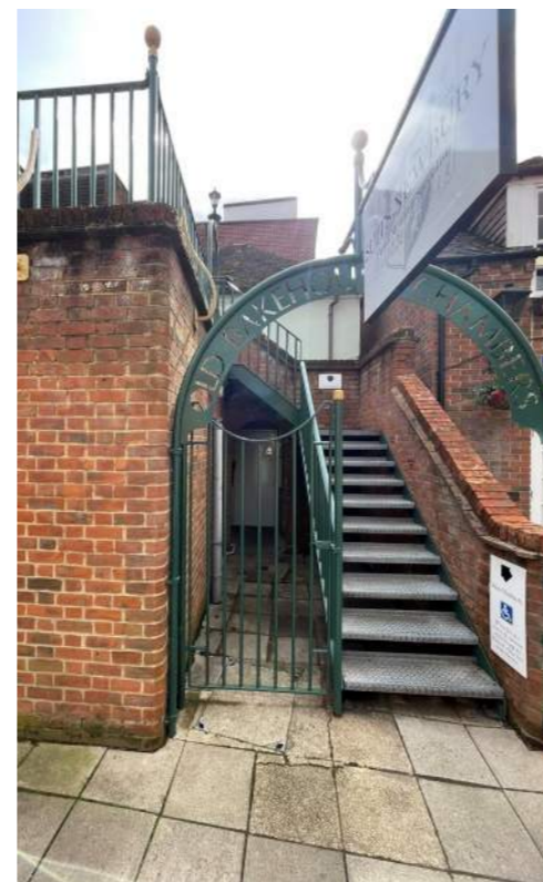
Figure 3.29: Weavers Walk metal stair access.
