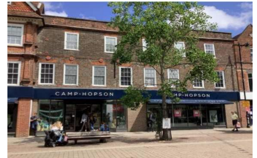
Figure 2.53: Northbrook Street. (Source: NTCAAMP).
