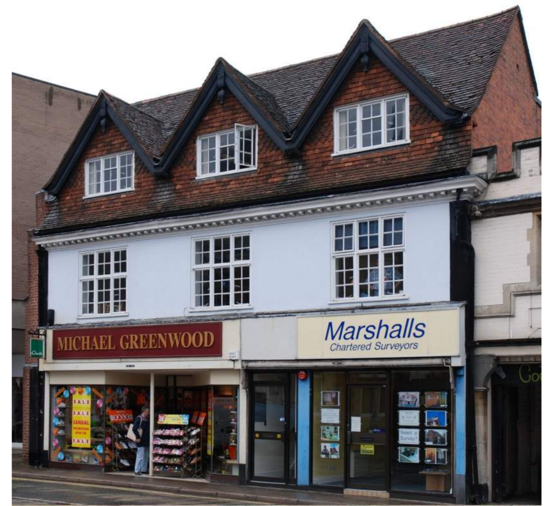
Figure 2.13: 33 & 34 Cheap Street. (Source: Historic England).
