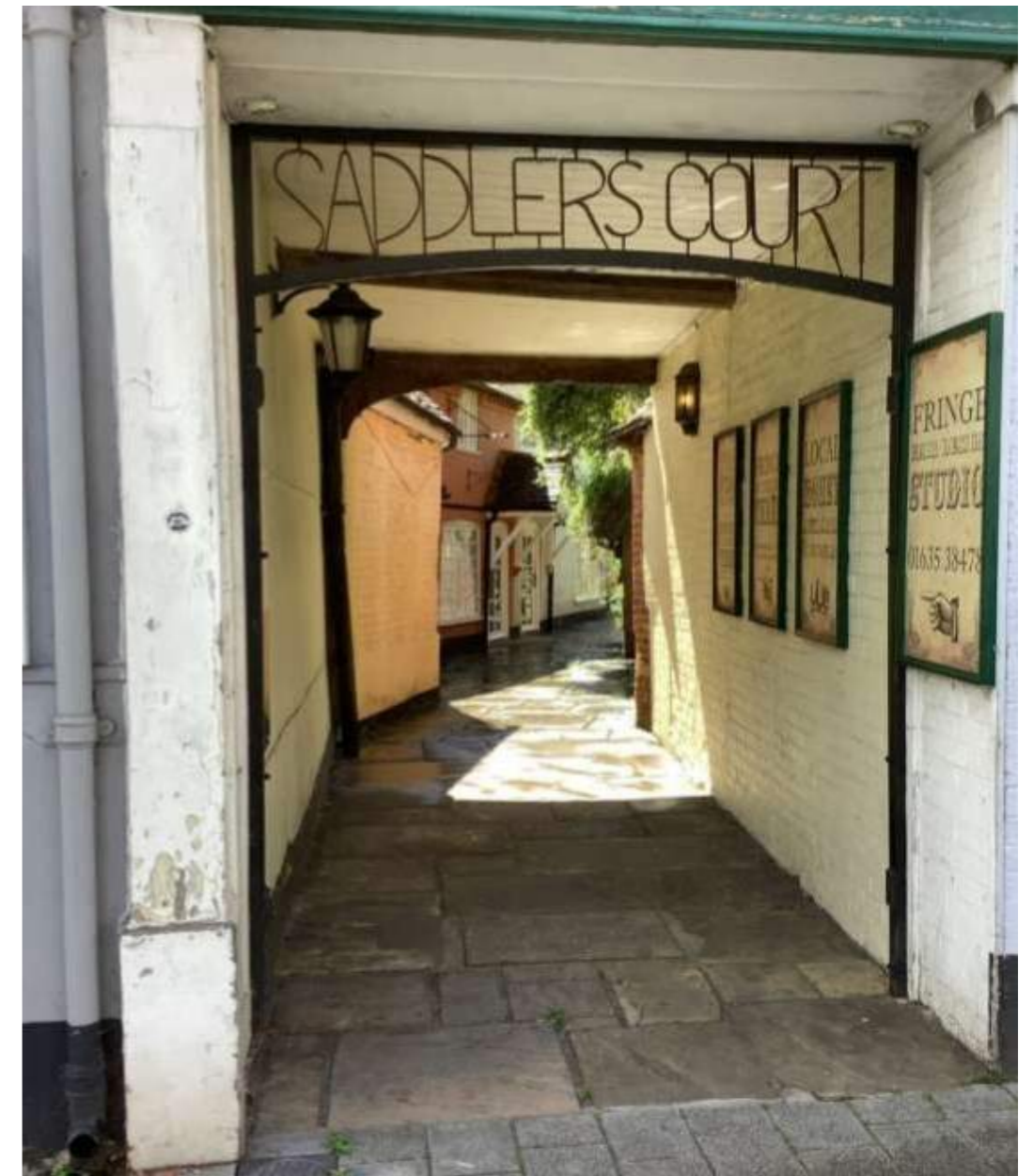
Figure 2.70: Saddlers Court - From Northbrook Street looking west, rich historic fabric is visible. (Source: NTCAAMP).
