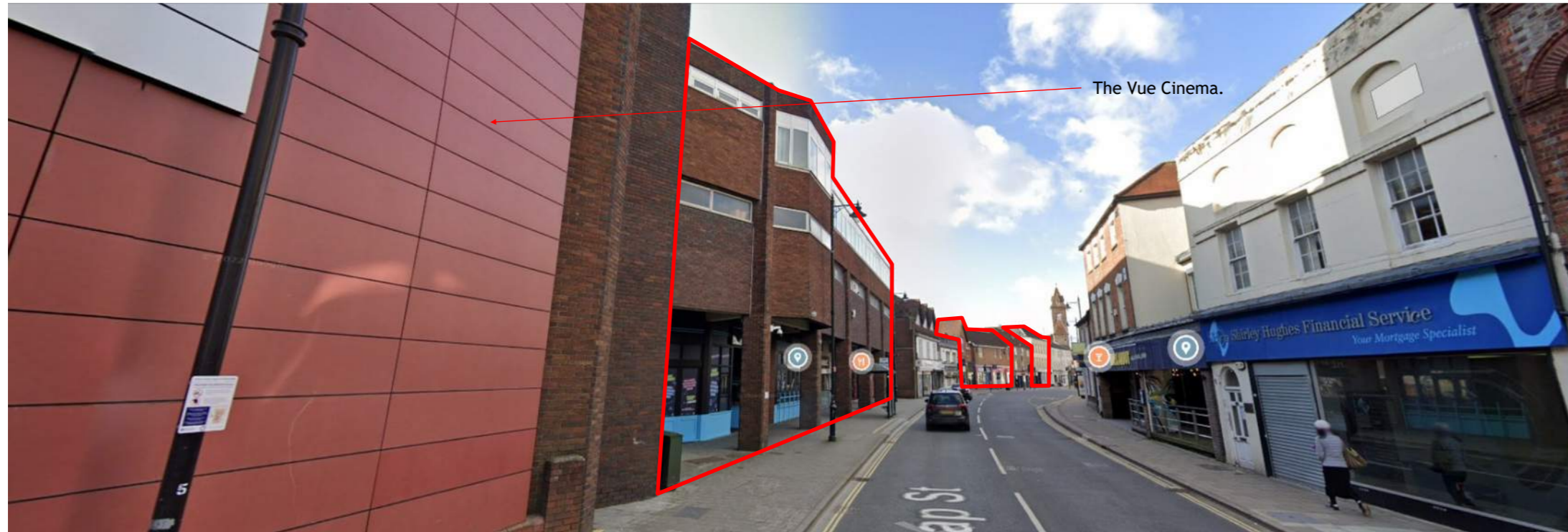
Figure 2.59: Cheap Street View - The buildings outlined red are the Negative, Neutral and one Positive Contributors proposed to be demolished as part of the Application.
