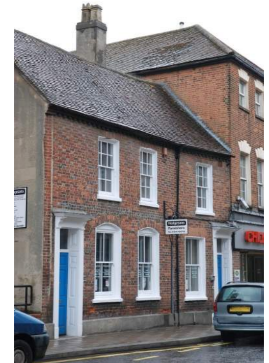
Figure 2.19: 41 Cheap Street. (Source: Historic England).
