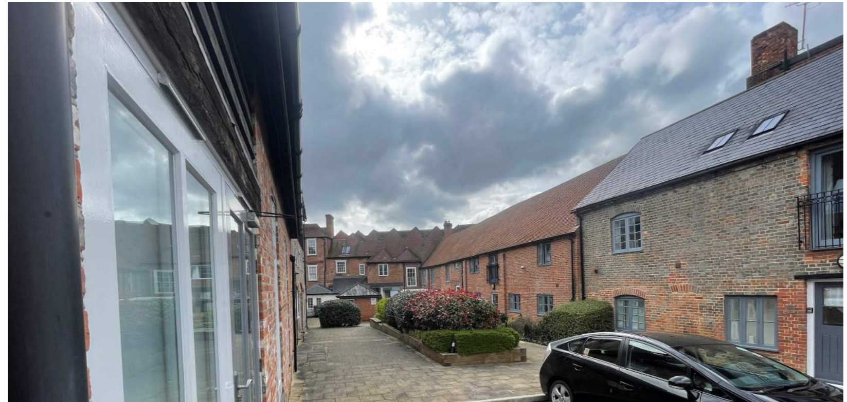
Figure 3.19: Outbuildings to the r/o 24 The Broadway (former Adnams Brewery) are on the left hand side with the outbuildings to the r/o 4 Oxford Street on the right frame the elevated linear courtyard space. In the centre is the raised planting bed.
