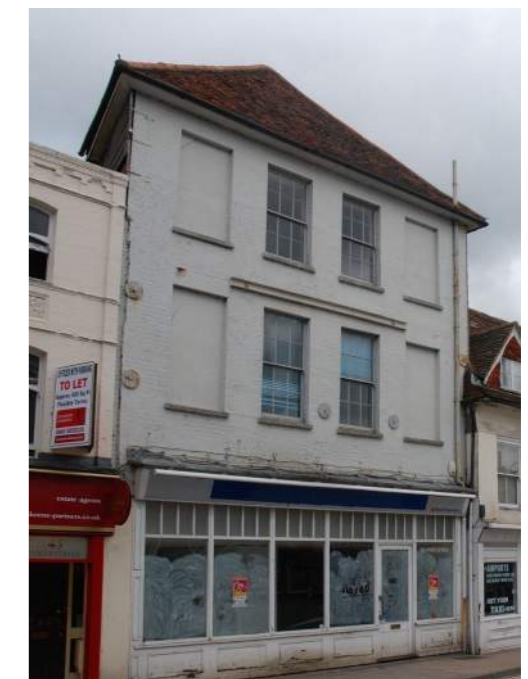
Figure 2.21: 48 Cheap Street. (Source: Historic England).
