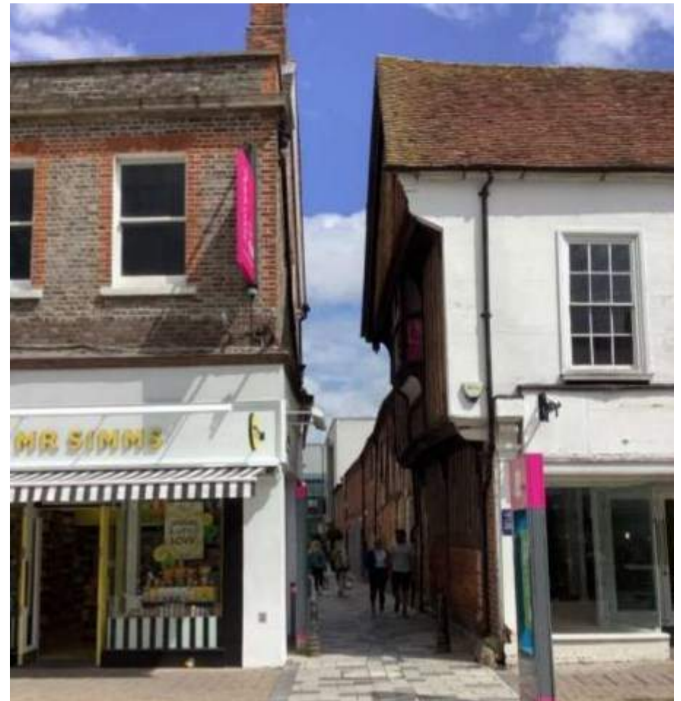
Figure 2.73: Marsh Lane - Inside the Conservation Area. From Northbrook Street looking east, provides a sense of the deep plot pattern, historic fabric is visible. (Source: NTCAAMP).
