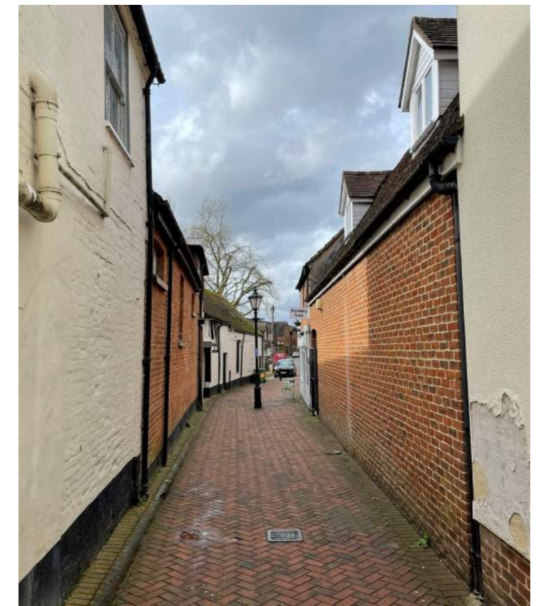
Figure 3.40: High-level windows offer daylighting into the buildings but protect the privacy from the passageway.
