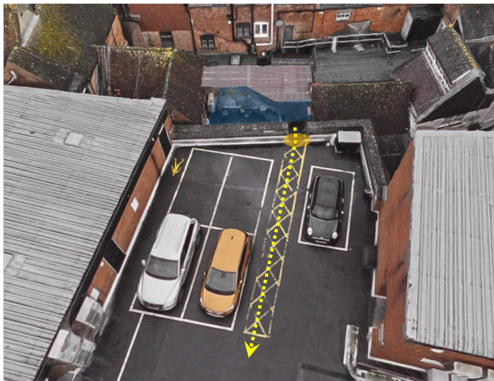
Figure 6.77: Existing Fire Escape route from The Globe Inn boundary across the Servicing Roof Top.
