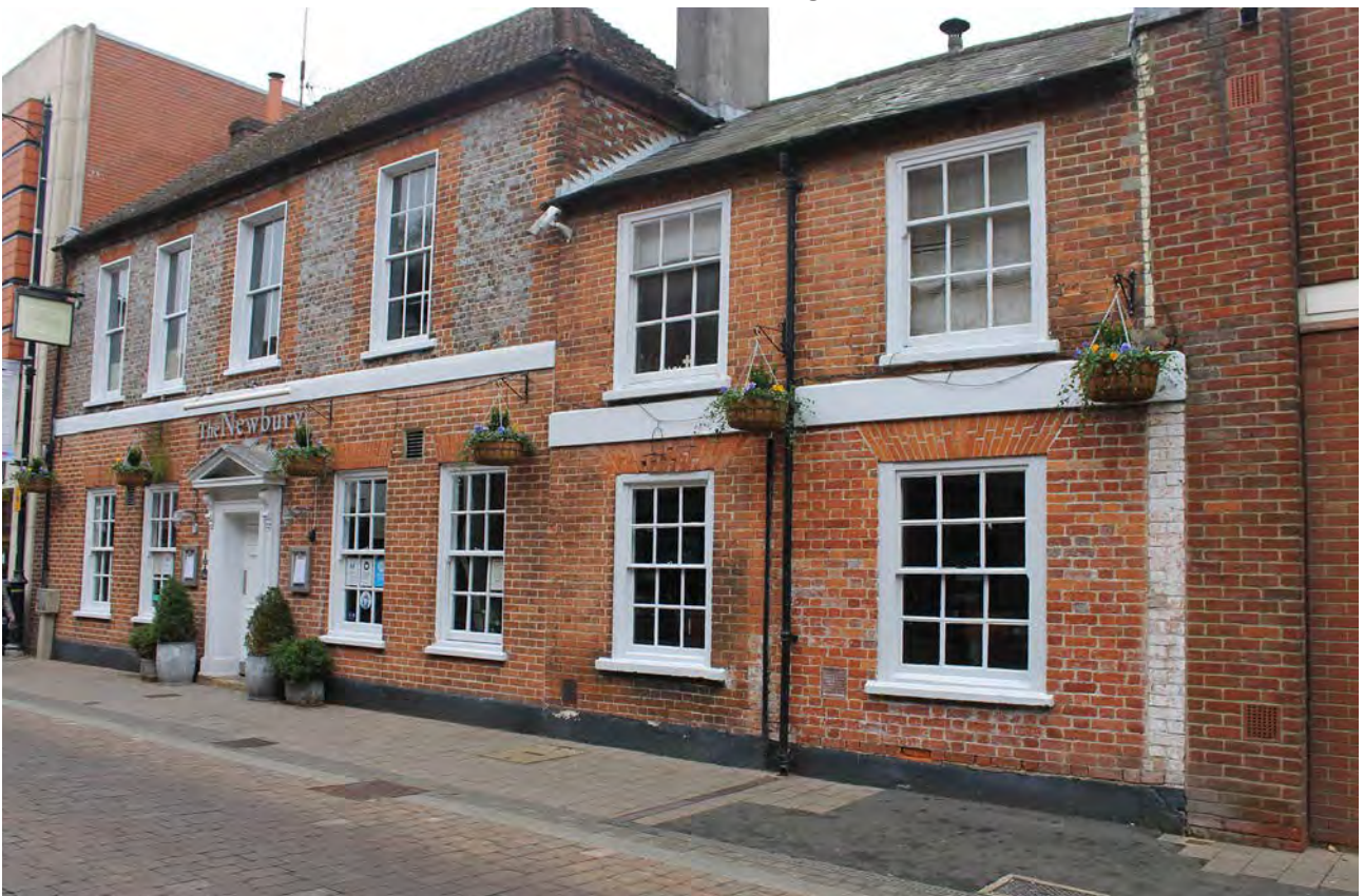
Plate 6: The Kennet Centre adjoining the Grade II listed The Newbury (formerly the Bricklayers Arms; OA 22), looking north-east
