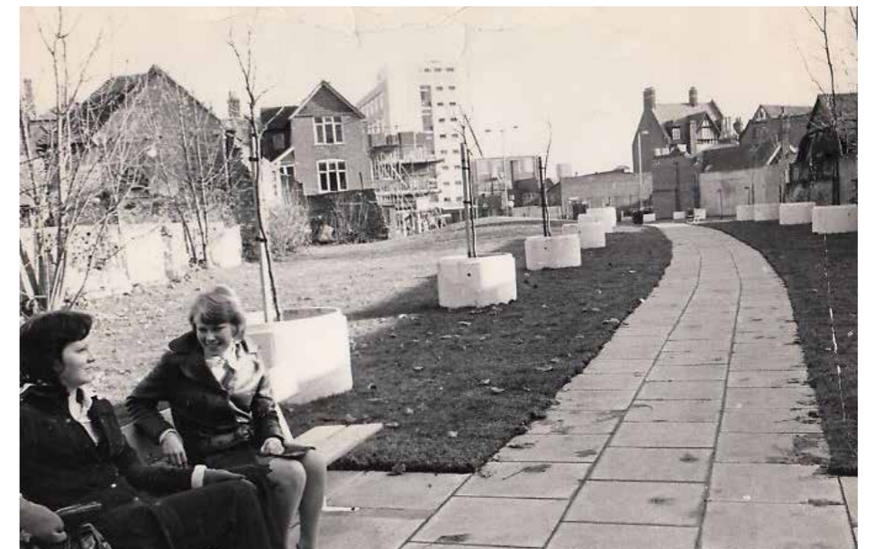
Figure 5.15 The building of the Kennet Centre, 1970s–80s
