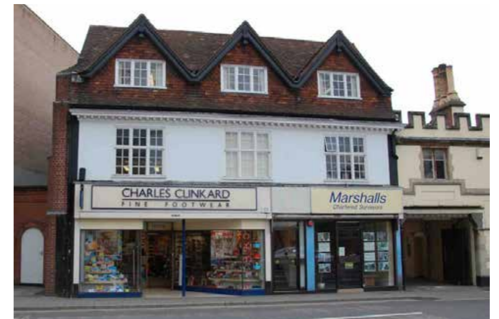
Figure 6.4 The Grade II 33 and 34 Cheap Street. Source: BritishListedBuildings.co.uk
