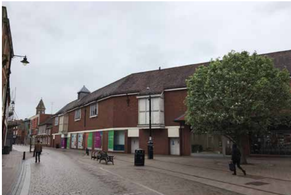
Figure 7.8 Inactivated façade of Kennet Centre along the south of Bartholomew Street.
