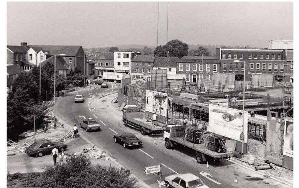
Figure 5.14 The building of the Kennet Centre, 1970s–80s
