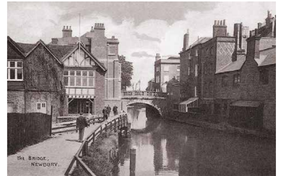
Figure 4.5 Bridge over the River Kennet at Newbury, 1904
