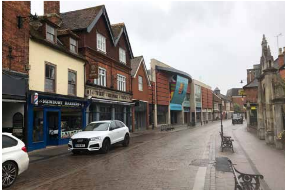
Figure 7.7 Inactivated façade of Kennet Centre along the north of Bartholomew Street.
