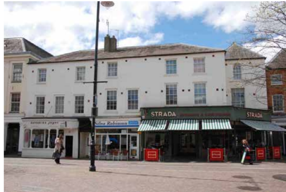
Figure 6.5 The Grade II listed 21-25 Market Place. Source: BritishListedBuildings.co.uk.
