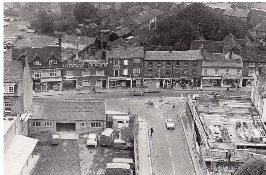
Figure 5.13 The building of the Kennet Centre, 1970s–80s
