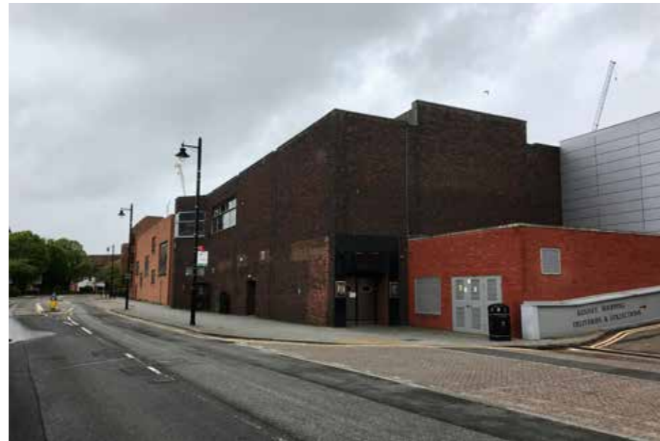
Figure 7.10 Inactivated façade of Kennet Centre along Market Street.
